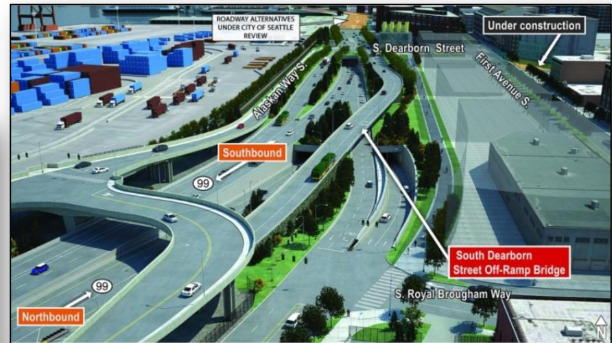
South Dearborn Street off-ramp (under construction)
