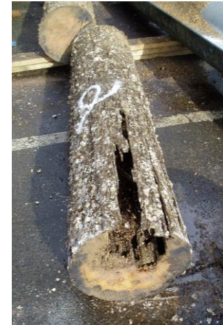
Timber pile that was removed and replaced due to deterioration
