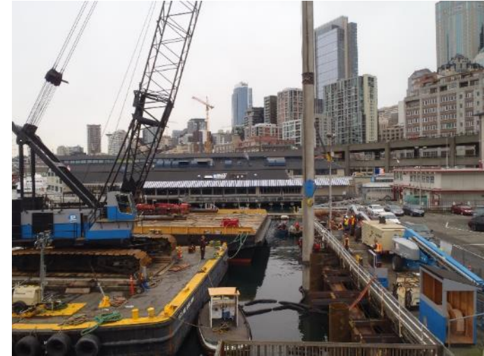
Hoffman-Pacific crews install a test pile at Colman Dock – January 2016
